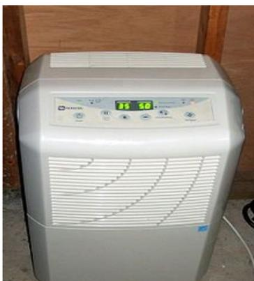
A dehumidifier is typically a household appliance that reduces the level of humidity in the air usually for health reasons. Humid air can
